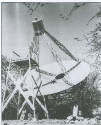
Fig. 3: Grote Reber's first antenna: a 31 ft. dish built in 1937. Photo: NRAO archives [11]
